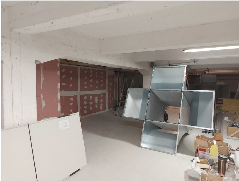
Figure 3. The anechoic termination before assembly
