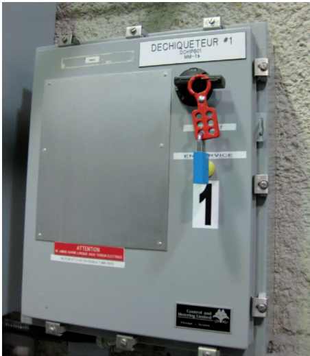
Figure 1. Individual lock applied on an electric isolating device.
