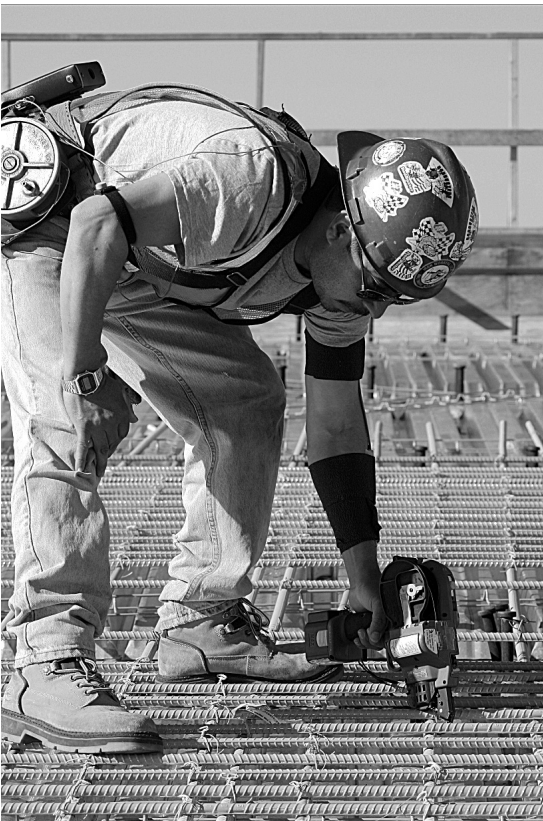
Figure 2. Tying rebar with power tier (PT).
